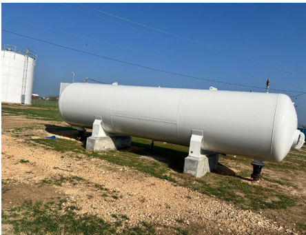
New 5k Gallon Pressure Tank
