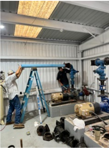
Piping & Valve Replacement Pump House
