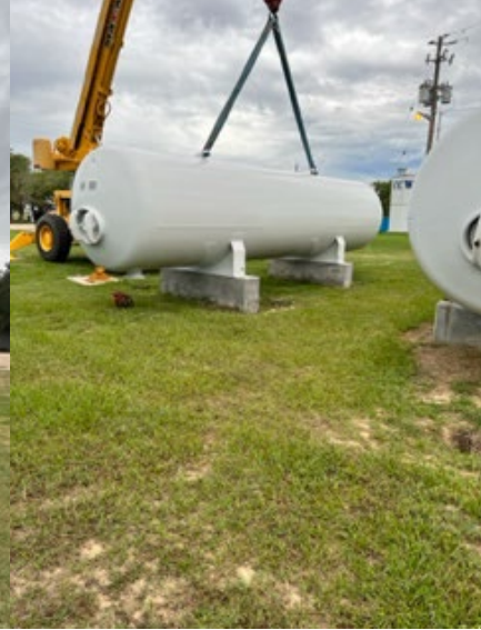
Placement of new 5k gallon pressure tank
