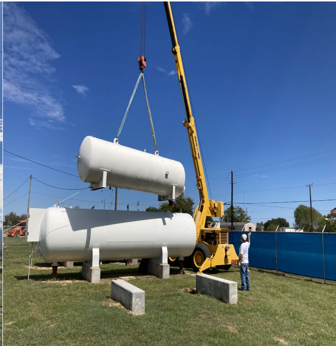
Removal of old 2.5k gallon pressure tank
