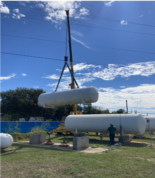
Removal of old 2.5k gallon pressure tank
